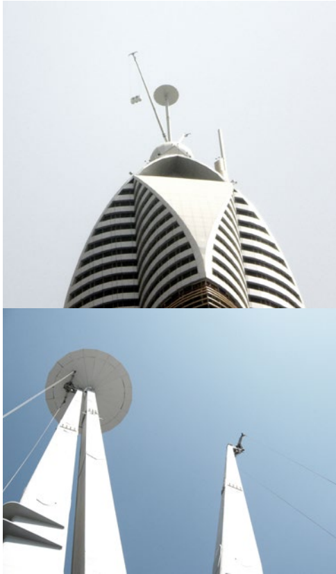
Rose Rotana Hotel, Dubai: Retractable crane BMU with twins jibs for optimal cleaning service
