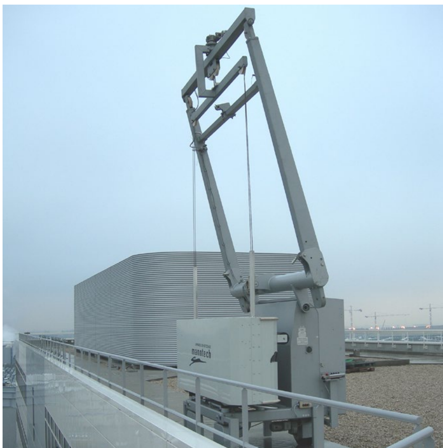
Type 1.3 with crossbar for load-bearing hoist
