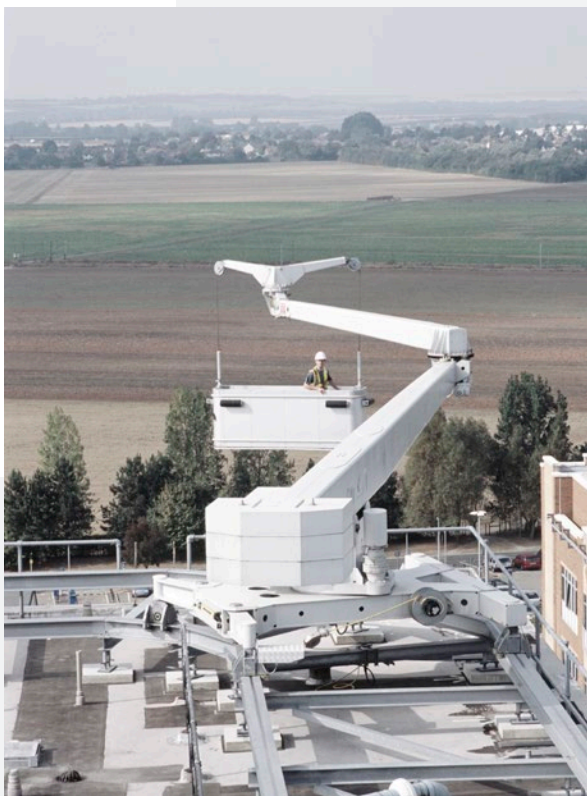
Type 6.1 track-based with horizontal slewing articulated jib
