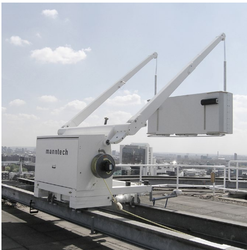
Type 1.1 with retractable jibs for parked position
